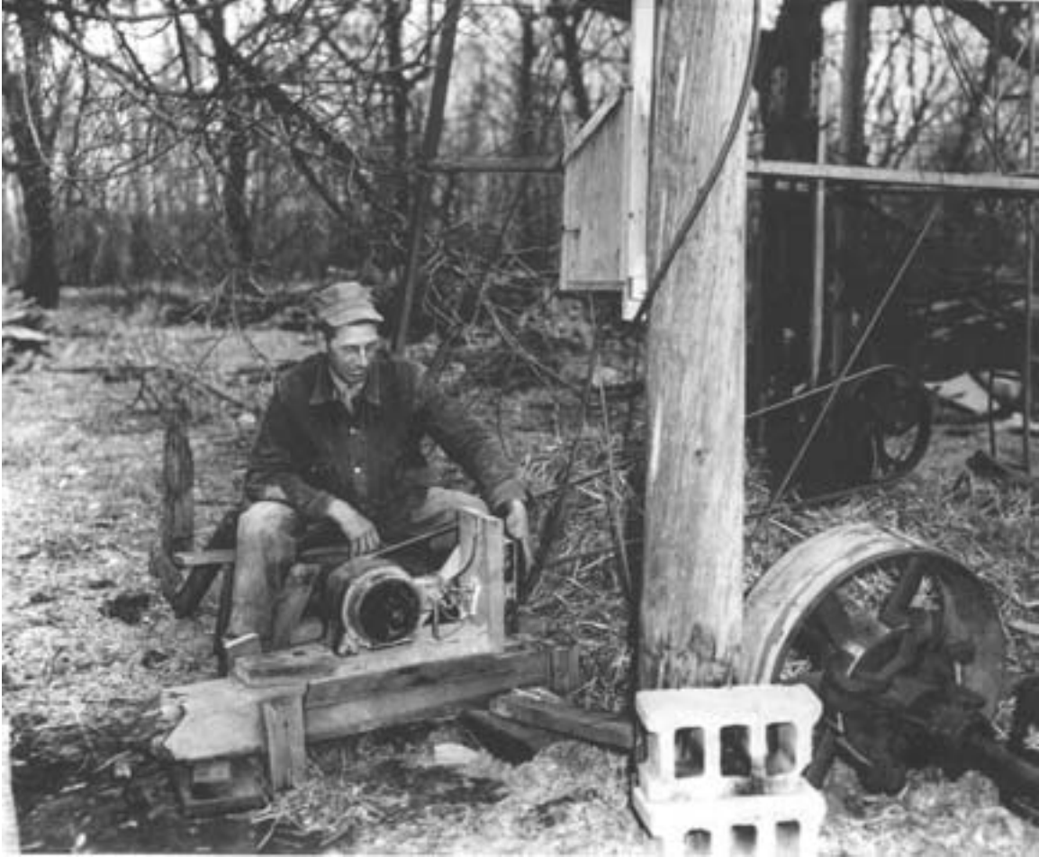
An electric pump being used near the base of a steel windmill tower. After farms electrified and modern water pumps were installed, windmills were eventually phased out. Location unknown, 1938. (MHS photo)
