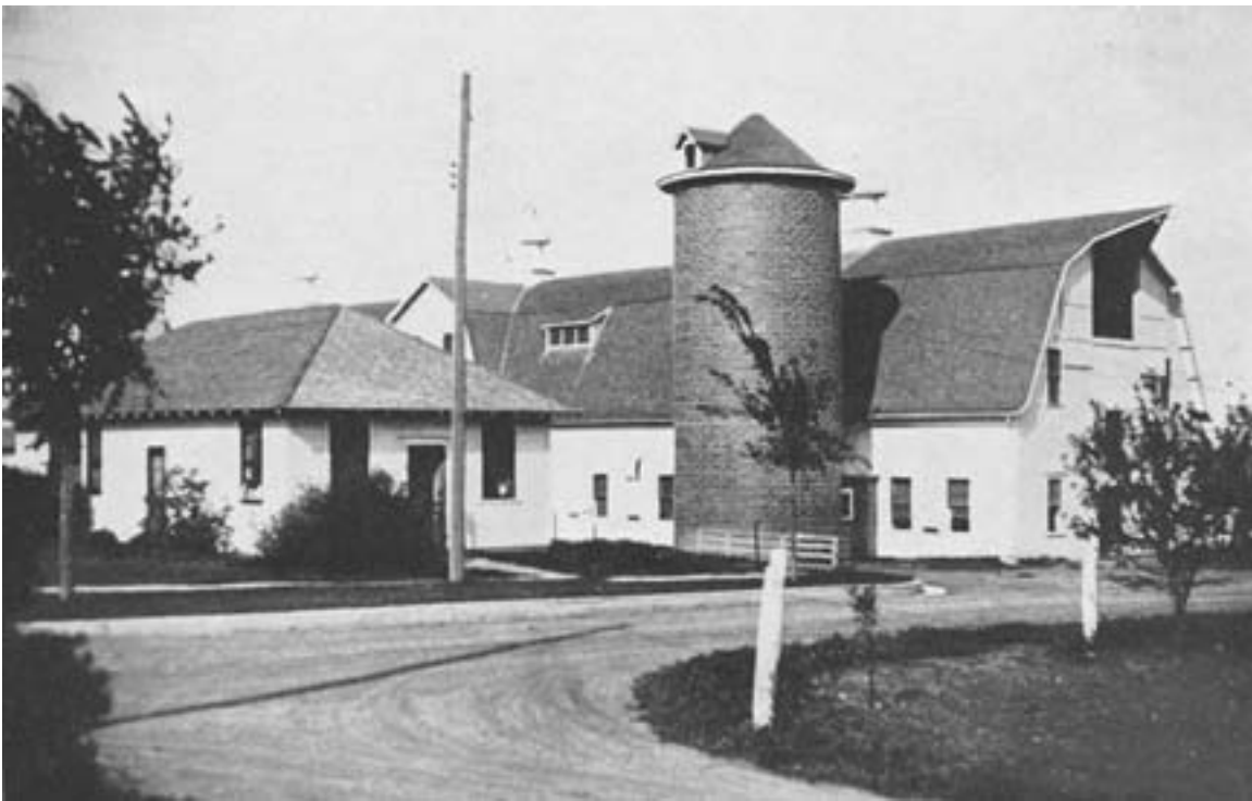
Dairy barn (1914), silo, and milk house at the West Central Experiment Station at Morris, which served 17 counties in western Minnesota. In an effort to get area farmers to diversify into dairying, Station staff distributed alfalfa seed and convinced farmers to build silos. One annual Visitors' Day in July of 1920 drew 8,000 to 9,000 people to the station to examine test plots and buildings, attend demonstrations, and socialize. Circa 1926. (West Central Minnesota Historical Research Center photo)
