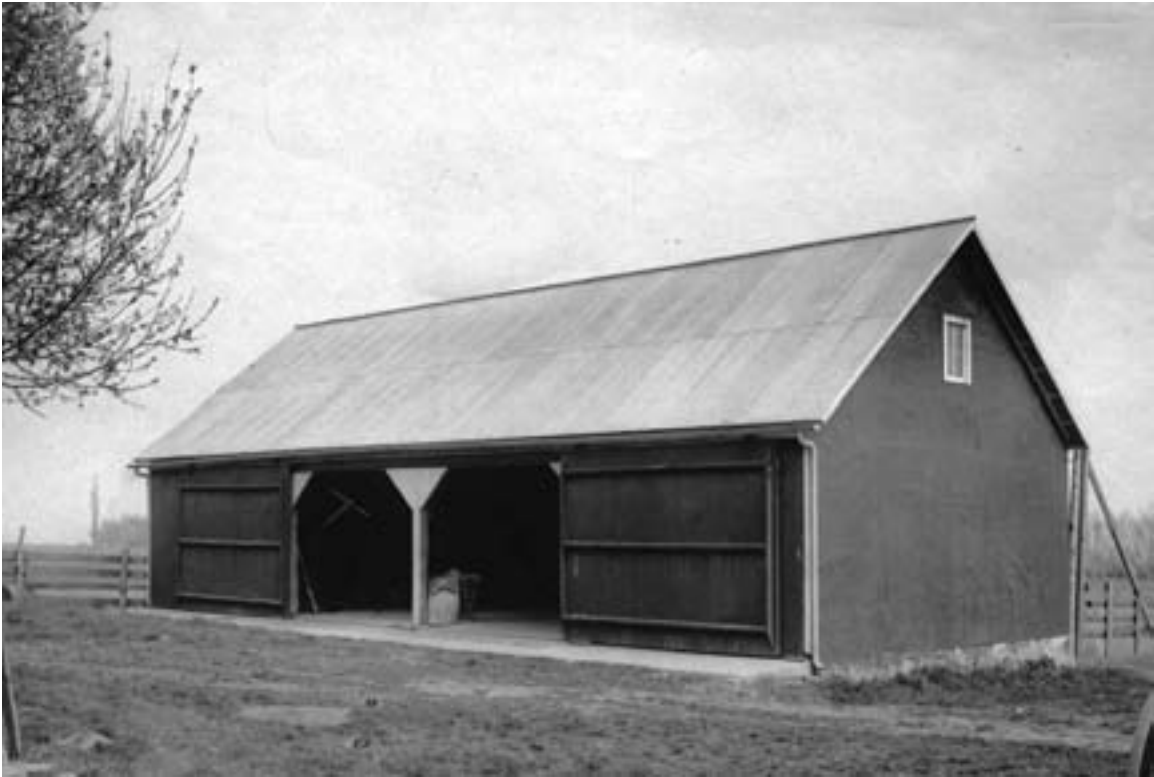
An implement or machine shed with sheet metal siding and roofing, and a sliding door. Location unknown, circa 1910. (MHS photo by Harry Darius Ayer)
