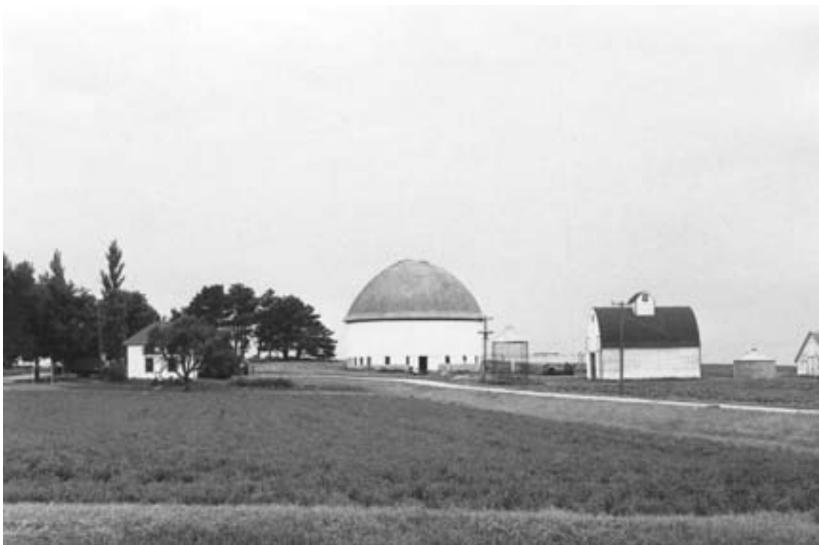
This farm's electrical transmission line is coming in along the driveway. Near Rapidan, Blue Earth County, circa 1972. (MHS photo)
