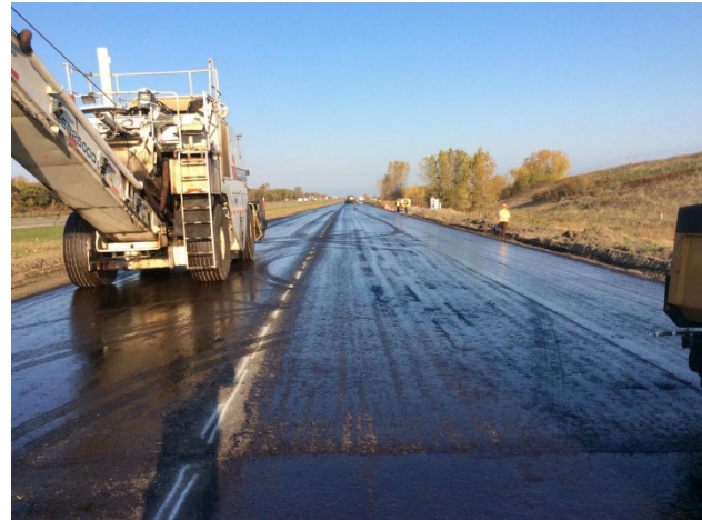
Figure 1.1-2 - Tack coat application at MnROAD 2016.
