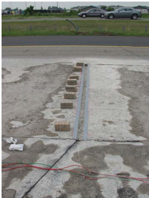
PIEZO QUARTZ SENSOR INSTALLATION
