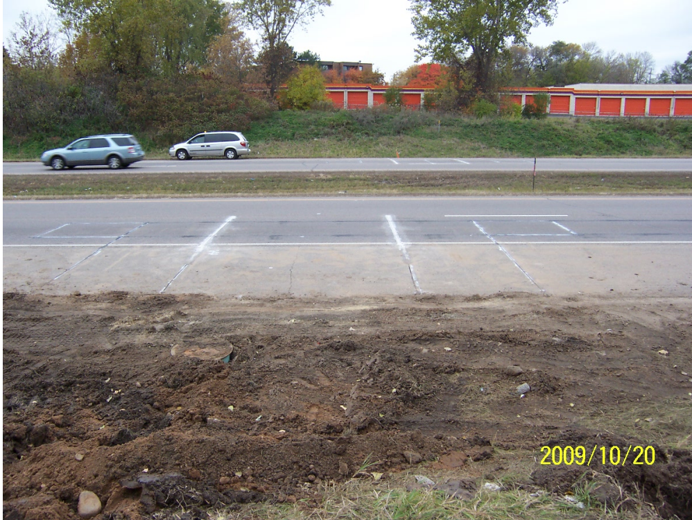
Figure 2. Typical WIM Site Lane Sensor Layout (Source: MnDOT files)
