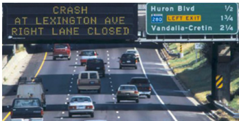
Dynamic Message Signs Source: 2014 MnDOT ITS Manual
