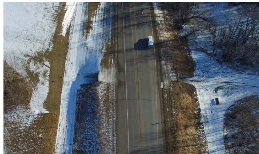
Figure 2.23: Underpass Crossing at 1,000 feet east of TH 29/Manor Hills Intersection
