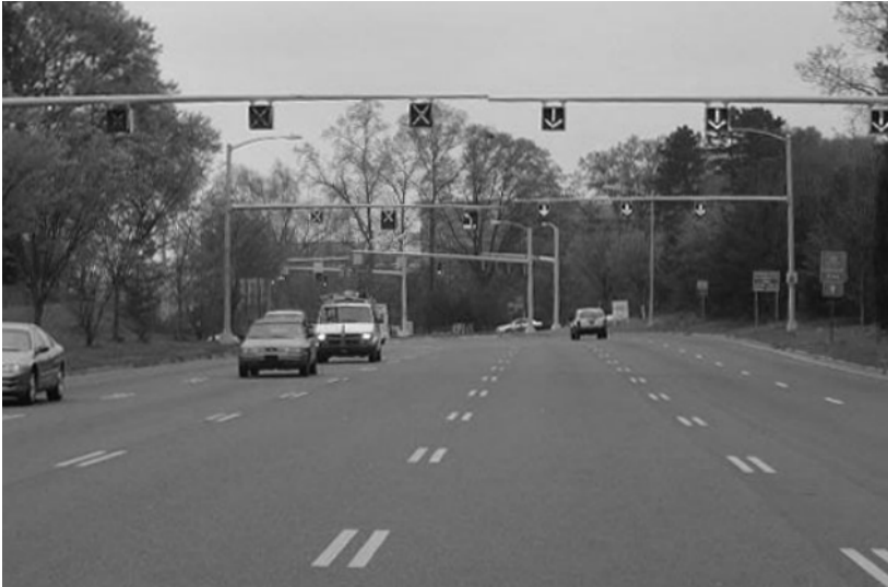
Figure 3.17: Example of Reversible flow lane segment (Section of Tyvola Road in Charlotte, NC)
