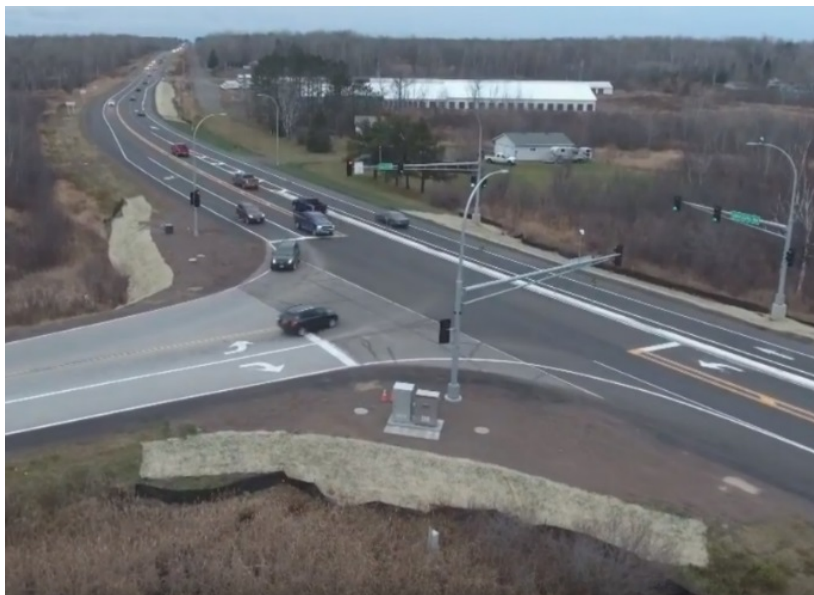
Figure 3.9: Example of a typical Green T-Intersection (CSAH 4 & Airport Road in Duluth, MN)
