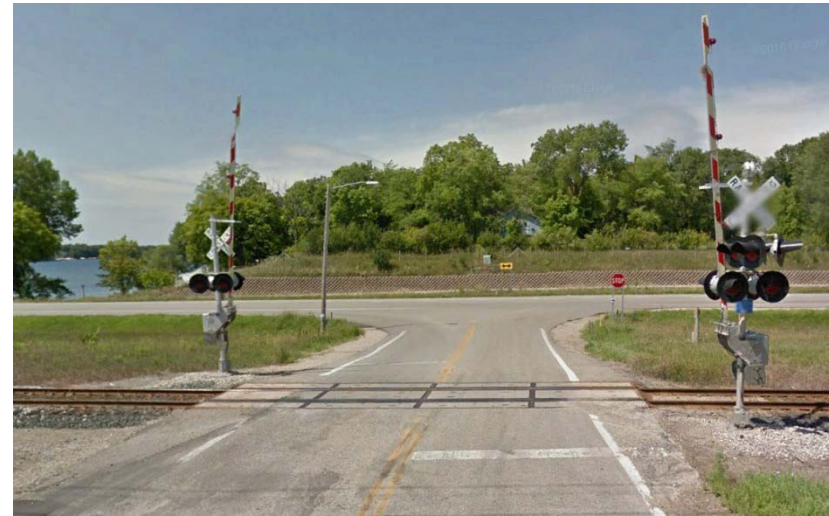
Figure 2.25: Railroad Crossing- facing TH 29 roadway (Google Earth)
