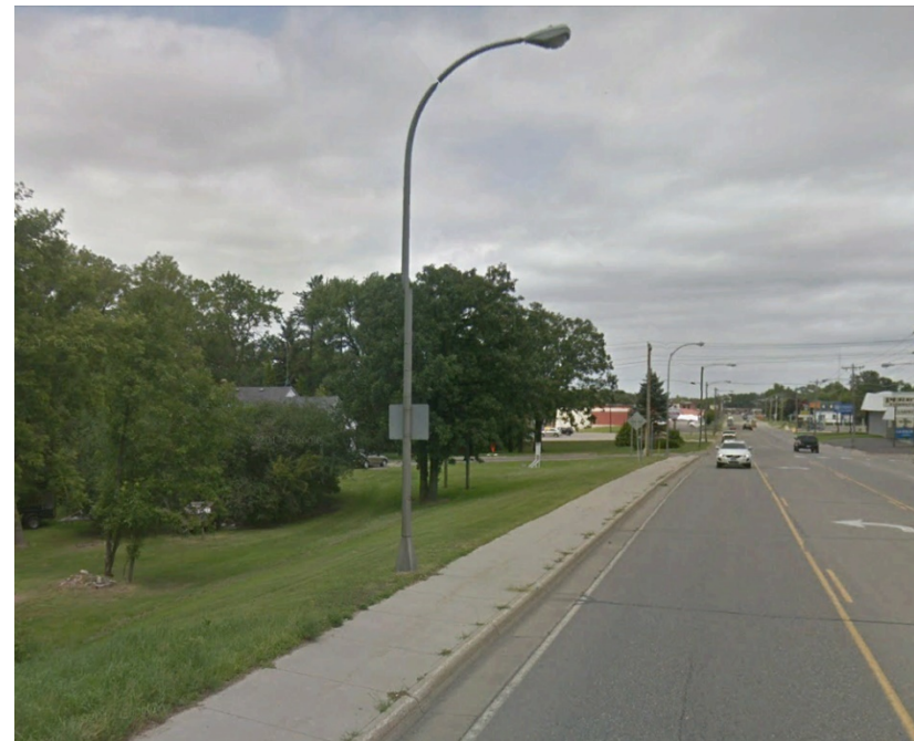
Figure 2.20: Light Poles Installed in Boulevard (Google Earth)
