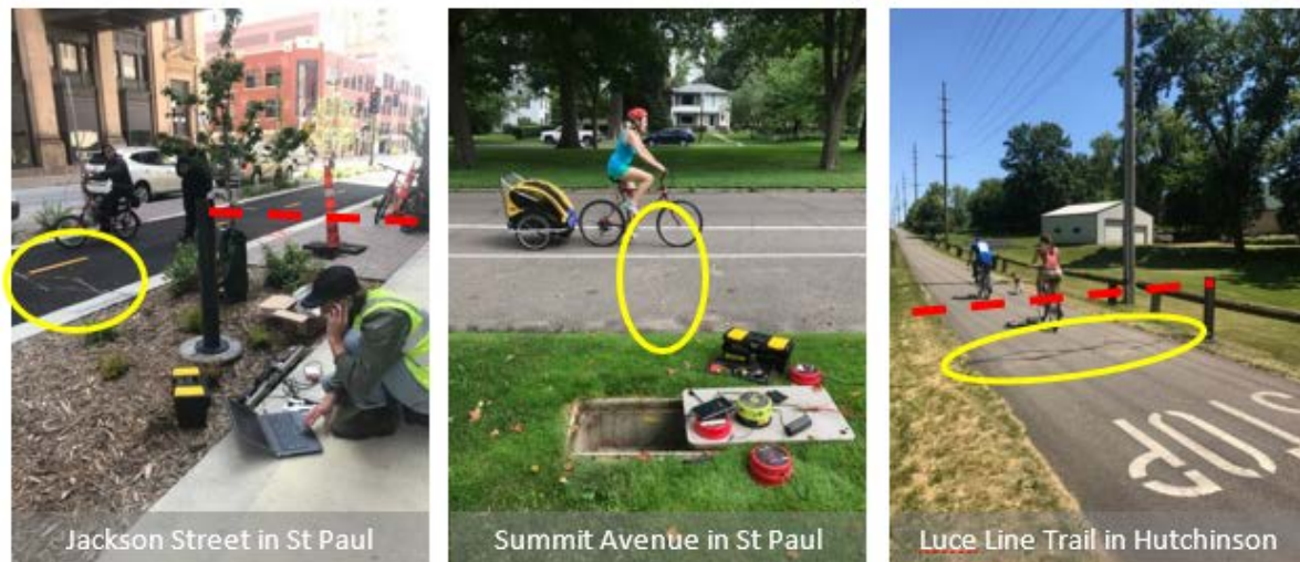
Figure 2: Different types of permanent installations (red dashed line indicates passive IR sensor and the yellow ovals identify inductive loops).
