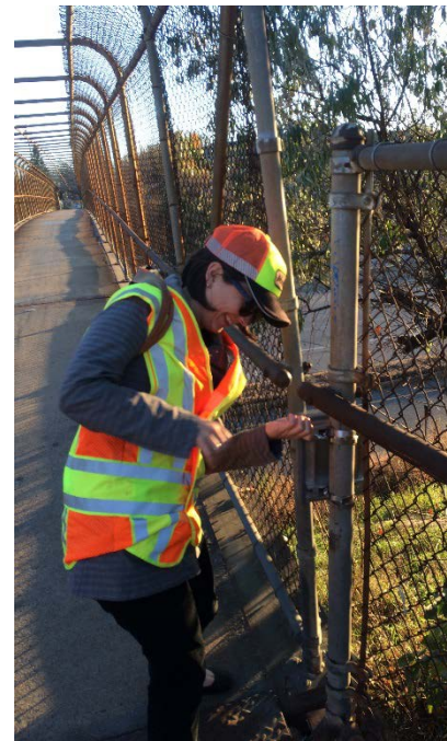
Figure 15: Installation of a portable Pyro (passive IR) counter.
