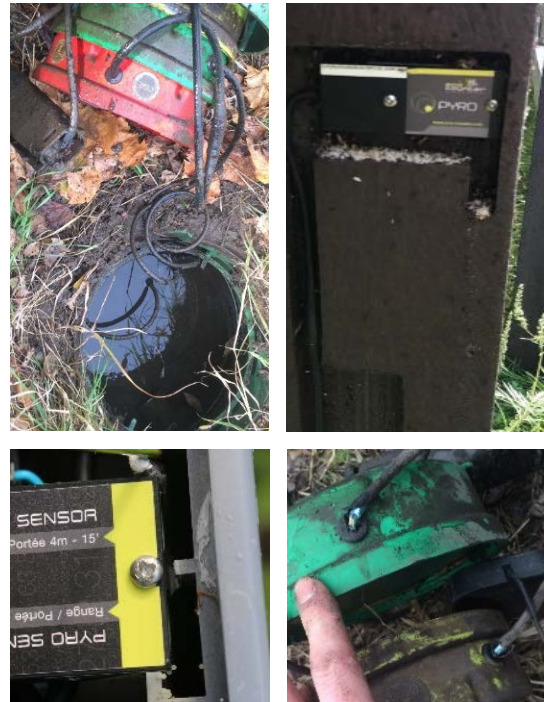
Figure 3: Examples of environmental and equipment issues. Clockwise from top left – water infiltration, ant infestation, cracked cable housings, spider web with eggs.
